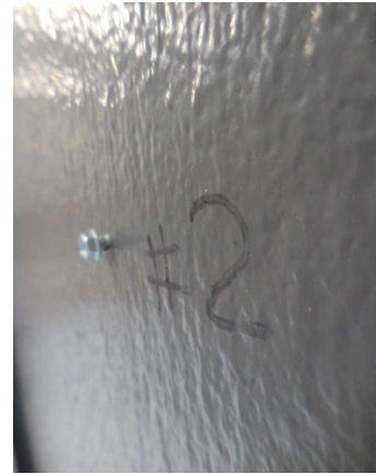
Close up of fastener
