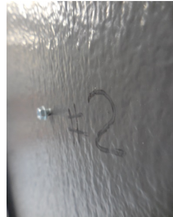
Close up of fastener
